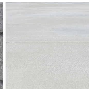
CONCRETE SEALER On Concrete Flooring
